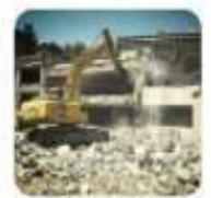
Urban Transformation Building Demolition Service
